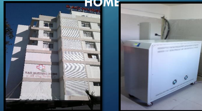
125KVA x 2 nos. ONLINE UPS for CATH LAB machine at RAO NURSING HOME
